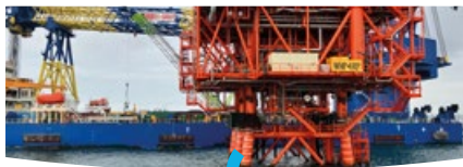
Fiber Optic Monitoring Republic of Congo
