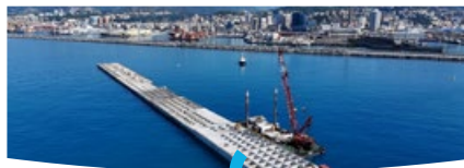
PerGenova Breakwater Genoa, Italy
